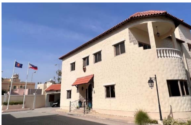
One of the four villas comprising the new PHL Chancery in Adliya, Kingdom of Bahrain
